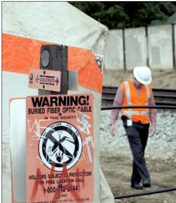
A sign warns that buried communications cables are present next to the underground vault where police suspect vandals entered and cut several of the lines in San Jose, Calif., on Thursday.
