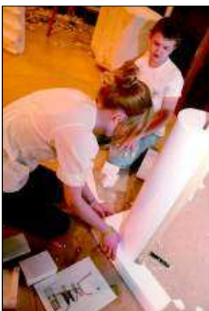
Twin Falls High School student Catina Crum works with classmate Dalton Mortensen in building a stage which features columns — a Spanish architectural flourish for 'Bernarda,' set in Spain.
