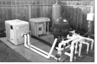
Photo courtesy of ClearWater Tech An ozone pool purifier system is connected to the pool plumbing system.
