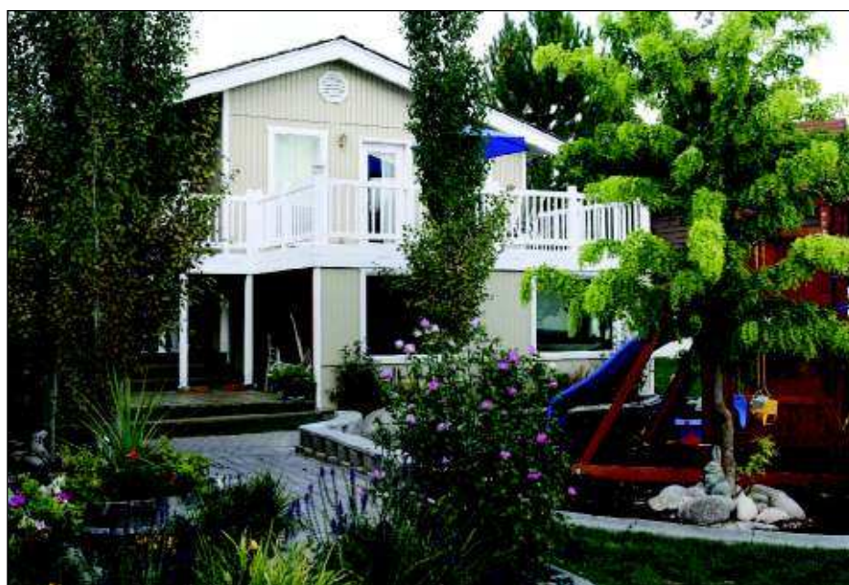
The Votroubeks' new deck is seen from the yard. The existing second-floor deck was too dangerous to use and had no access from ground level.
