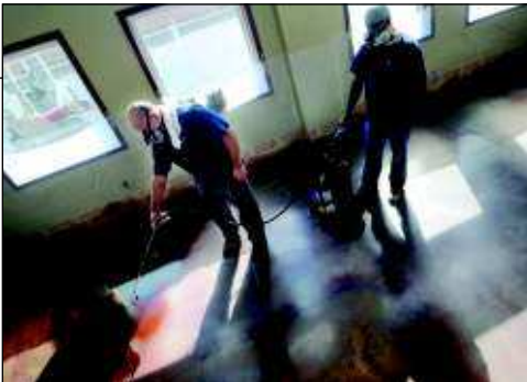
MCT photo Jeremy Williams, left, and Isreal Carbajal use red dye to create a stained concrete floor in Tacoma, Wash.
