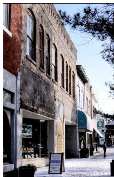
The building at 120 Main Ave. N. in historic downtown Twin Falls looks completely different without the yellow, tin siding that covered the original masonry work and windows on the second story. A grant awarded to the Twin Falls Historic Preservation Committee paid for an architectural study that determined if the tin could be removed and what needs done to rehabilitate the front.
