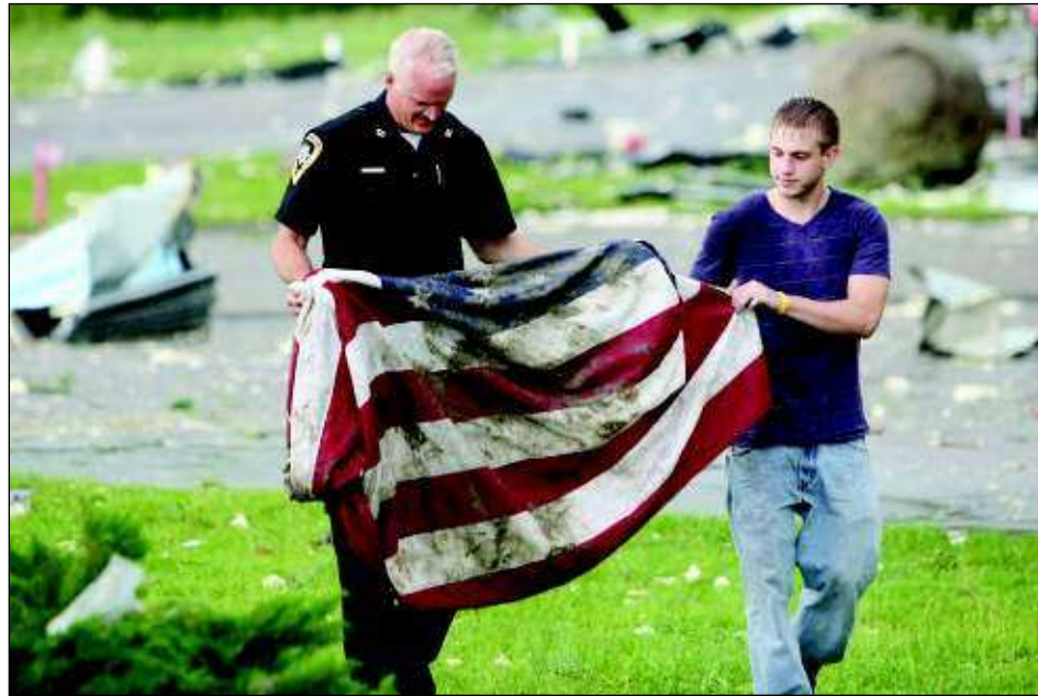
Sheriff Deputy John Smith and Taylor Brown find a flag that was found near the Rimrock Auto Arena at MetraPark in Billings, Mont., after a tornado extensively damaged the 12,000-seat facility on Sunday.
