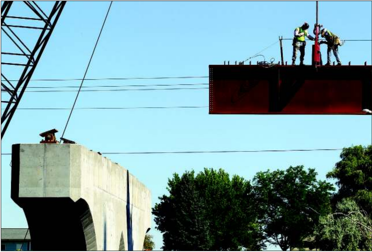
OlsenBeal Construction workers crank down an I-beam clamp while installing the first of 21 girders for a bridge over the Rock Creek Canyon, as part of the Idaho Transportation Department's Twin Falls Alternate Route project Monday east of Twin Falls. After wind prevented the work last week, crews were able to move ahead with the bridge installation that is part of the $26.6 million federally funded project.
