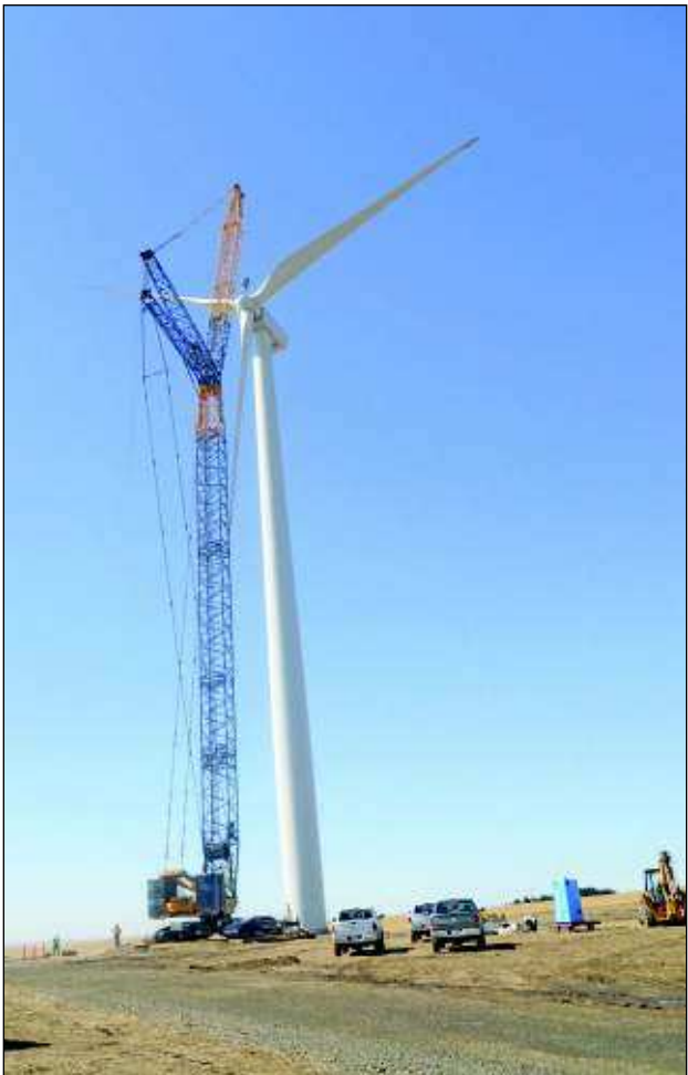
AP photo A crane hoists up blades to install in the first of six wind turbines at a Wind Farm near the southern border of Idaho and Oregon.
