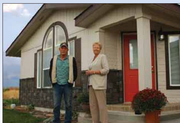
With the help of family members, Harlan and Debbie Wensink redid the exterior of their Gooding home with faux rock tiles, new paint, light fixtures and a tiled front porch.
