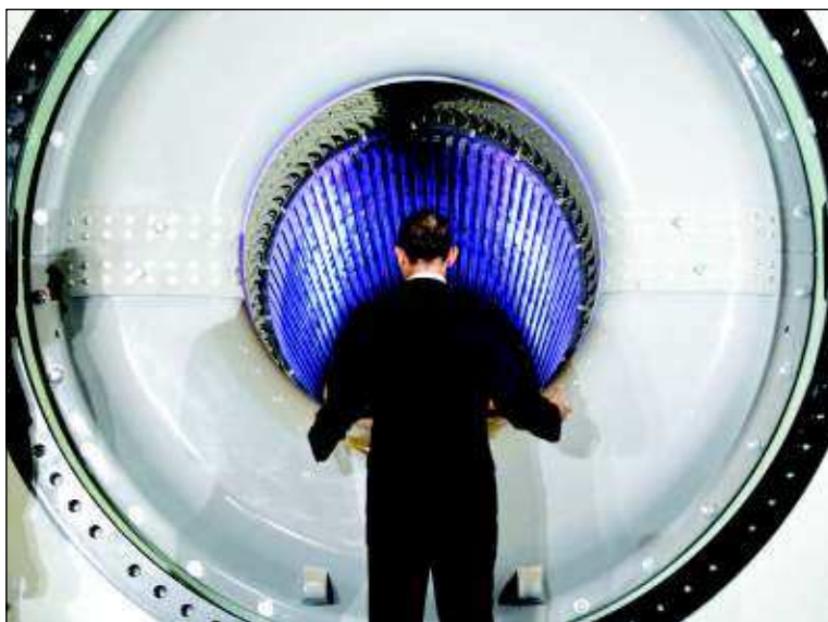
President Obama peers into a hydro-gen-cooled generator being made for a power station in Kuwait as he tours a GE plant in Schenectady, N.Y., to talk about clean energy and green jobs on Jan. 21.
