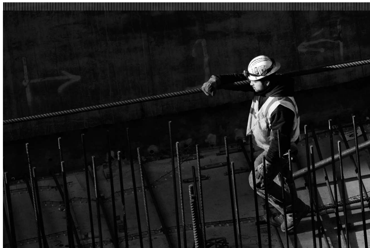
On Dec. 29, a construction worker carries a steel bar for the foundation of 3 World Trade Center in New York. The eighty story office tower is one of three skyscrapers at the site under construction by developer Silverstein Properties. U.S. builders spent more in November on single-family home construction, apartment building and remodeling projects, pushing construction spending up by the largest amount since August.
