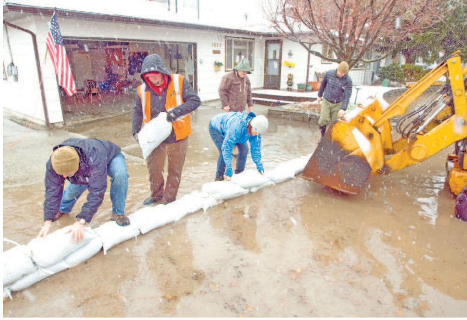
AP PHOTO • MOSCOW-PULLMAN DAILY NEWS, GEOFF CRIMMINS Residents and city employees stack sandbags outside a home at the intersection of Hillcrest and Bridge streets, Monday in Moscow. Paradise Creek was flooding the neighborhood.
