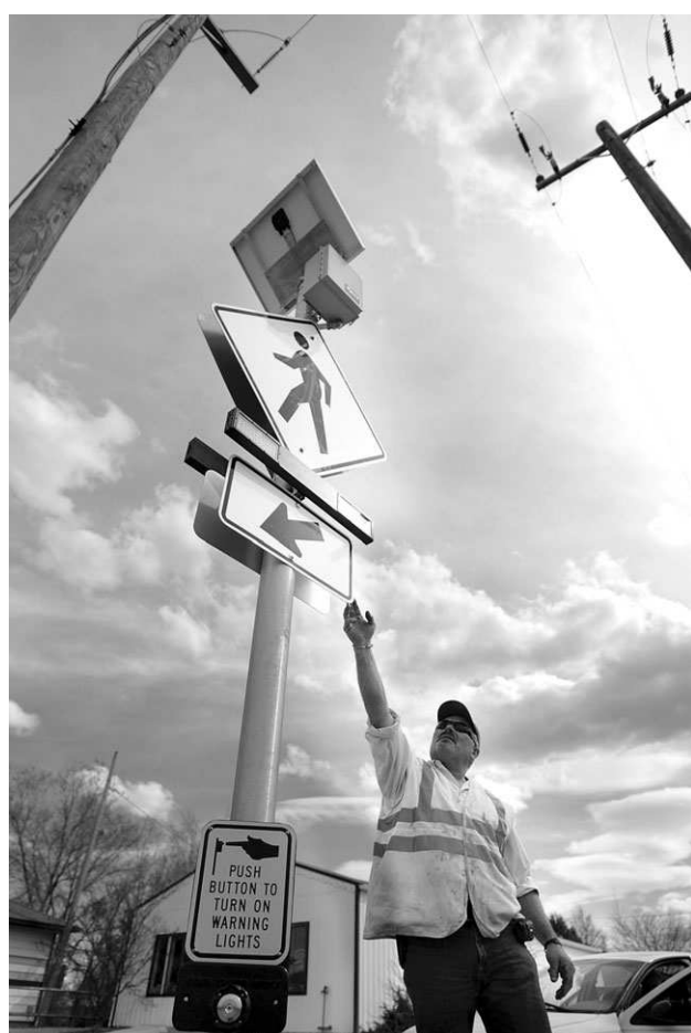
DREW NASH • TIMES-NEWS Terry Williamson, signing and striping coordinator for the city of Twin Falls, adjusts a new crosswalk warning light along Addison Avenue Tuesday.
