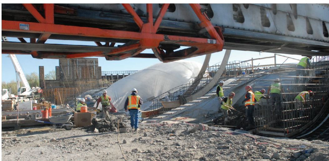
Crews work Thursday on a portion of the spillway designed in an S shape to accommodate the water flows. This portion of the spillway is 300 feet wide and 50 feet deep, and will have 12 gates.
