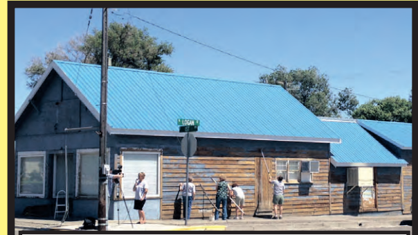
Glenns Ferry - KRUGER BUILDING – Before
