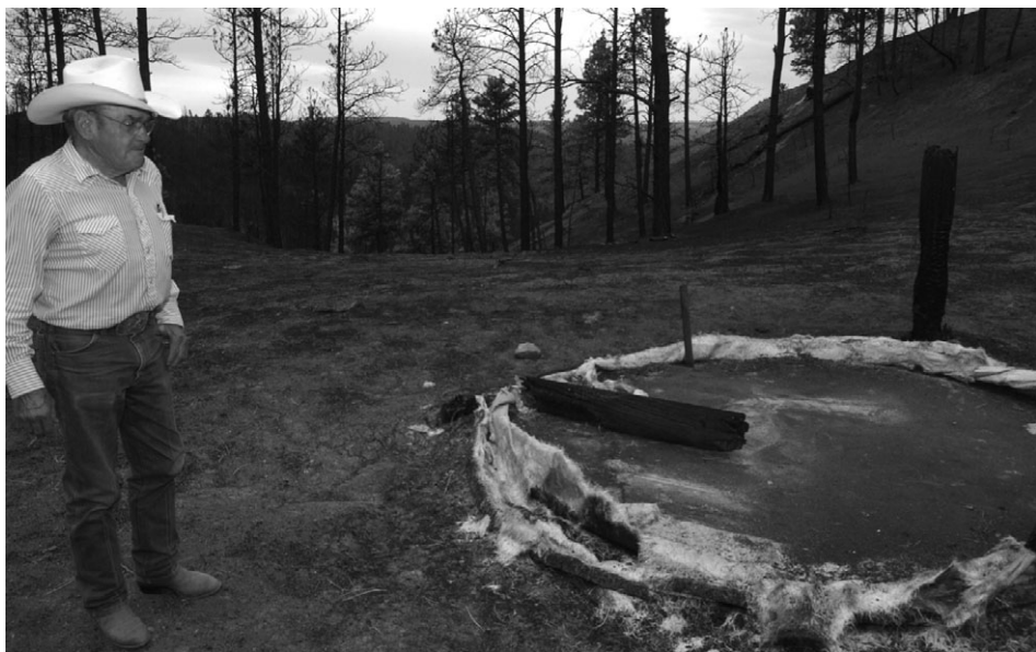
Cecil Kolka examines the remains of a fiberglass water tank July 20 in the Custer National Forest that melted during the Ash Creek Fire.
