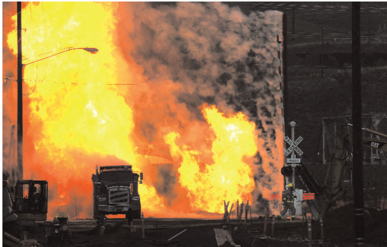
A towering column of flames rises into the air above Fifth Street in downtown Lewiston on Monday after an excavator hit a gas line.
