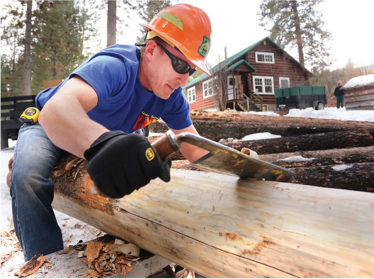
Bitterroot National Forest facility engineer Zac Hiedeman works to peel one of the logs that will be used to rebuild the front wall at the historic West Fork Ranger House on Tuesday in West Fork, Mont.
