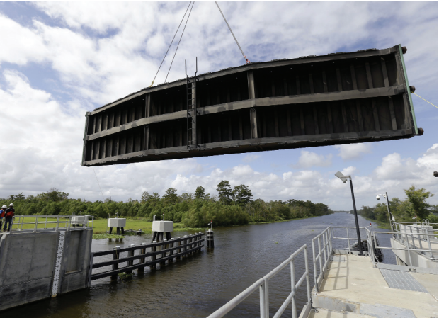
A crane lowers a flood gate into Hero Canal, as part of the hurricane protection system protecting the greater New Orleans area, in anticipation of Tropical Storm Karen, in Belle Chasse, La., Friday.
