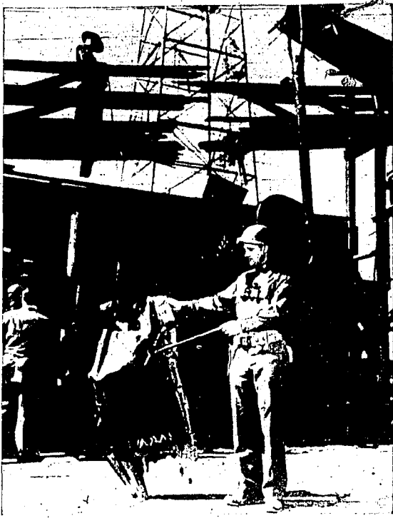
While the hunt continued by sea and air for the submarine which shelled the Ellwood, oil field and Hanklin refinery near Sacto, Harlan, Calif., a soldier surveys some of the damage wrought by the shell blast. He holds a sheet of metal perforated by a near miss of one of the raider's shells while above is a damaged oil well catwalk which suffered a direct hit.
