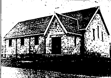
St. Paul's Lutheran church, Jerome, will be dedicated today to climax an unusual building program that saw the members of the congregation do the actual work and supply funds for needed articles and furnishings. (Times-News Photo and Engraving)
