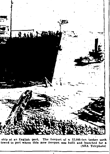
Novel launching was title of half a ship at an English port. The forepart of a 12,000-ton tanker sank after striking a mine. This part was towed to port where this new forepart was built and launched for "fitting."
