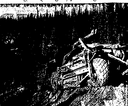
This mighty machine of peace, a tractor-drawn carry-all, helps build a wartime highway to Alaska through the forested Canadian wilderness. U. S. Army engineers constructing the road use this machine to move tons of earth from one section of the route to a fill.
