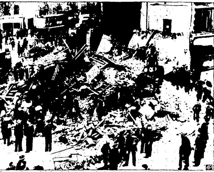
Rescue workers searched through the wreckage of a bank that was demolished in the German daylight air raid, the largest aerial attack on London since the battle of Britain. Picture radiated from London to New York.
