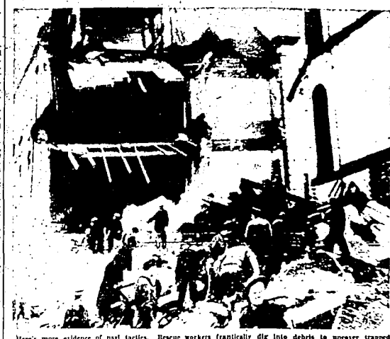
Here's more evidence of Nazi tactics. Rescue workers frantically dig into debris to unweaver trapped children in a London school building where the most recent German air raid Jan. 29 killed 20 pupils and injured 15. Photo Radio-News-Wire. (NEA Radio-Debris)
