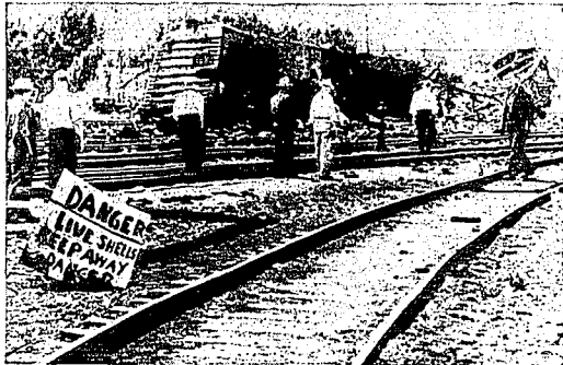
Here's the way the Grand Junction, Colo., railroad yard looked after two freight cars loaded with ammunition exploded and started firing all sizes and shapes of bullets and shells in every direction. The unscathed baggage, started from an overheated brake in one of the cars, injured but eight persons when one of the freight cars turned over on its side and the ammunition blasted in the opposite direction from the town's largest residential district.
