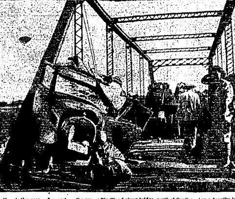
Here is a scene of a crash on the narrow bridge... The Blasec car was totally wrecked and the large truck severely damaged.
