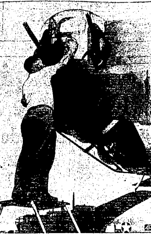
A formidable addition to Consolidated Valve Laboratory's armament is the Emerson electric turret being installed in the nose fuselage of the four-engine heavy bombers at Convair's Fort Worth, Tex., plant.
