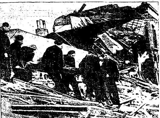
British workers carry an injured man from the wreckage of his home which was blasted by bombs dropped from German planes in their strongest attack on the British capital since the all-out bombings of 1941. Many homes were destroyed in this district. (AP wirephoto by Radio from London.)
