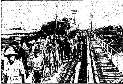
Foot traffic resumed across one of the bridges on Luzon island after it had been hurriedly repaired by U. S. army engineers. Retreating Japanese had destroyed the original span. Today's cables say the only thing that prevents General MacArthur himself from entering Manila is he had to turn back and await reports on a bridge near Manila that had been dynamited by the Japs.
