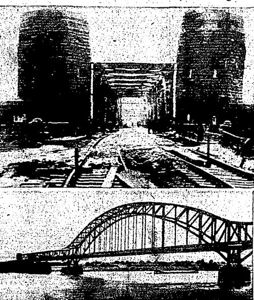
The views of the new famous Remagen bridge over the Rhine—once the Germans missed the boat for their westward escape, it was the only way to the east. The bridge was built by the U. S. Army Engineers and is now being used by the U. S. Army.
