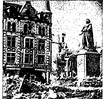
Music seems to have had a magic charm in the case of the state of New Jersey in the city square of Trenton, birthplace of the famous composer. Right next to it is debris of an air-raid shelter which received a direct hit during allied raid.
