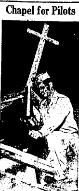
Chaplain Raymond Coleman, Cumberland, Md., helps with construction of a Chapel for Pilots.
