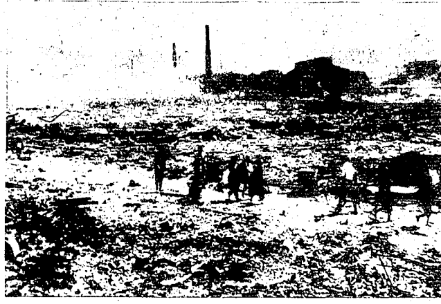
Japanese workers carry away debris in a devastated area of Nagasaki, Japanese industrial city on southwest Kyushu, after the Aug. 9 atomic bombing. Smokestacks and a lone building stand in the background. This picture, first ground view of atomic bombing damage, was released Sept. 1 by the army from files of Domei, official Jap news agency. (AP Wirephoto from U. S. Army signal corps)
