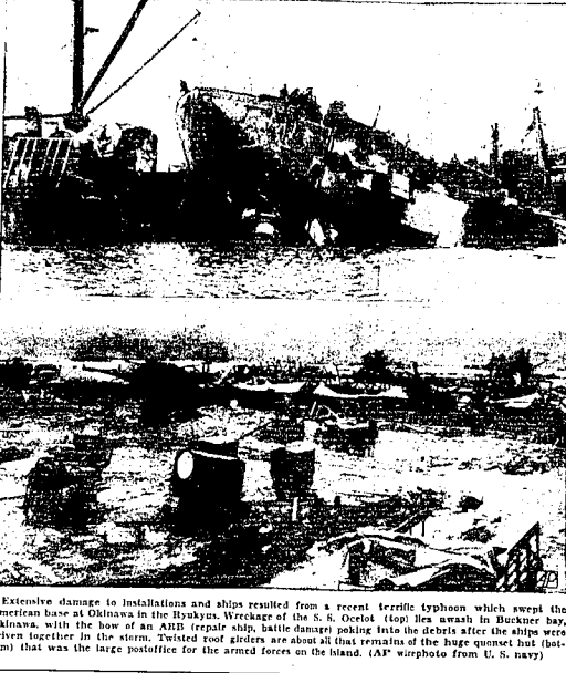
Extensive damage to installations and ships resulted from a recent terrific typhoon which swept the Okinawa. With the loss of an AHS transport ship, battle damage pointing into the debris after the ships were driven together in the storm. Twisted steel girders are about all that remains of the huge quonset hut (bottom) that was the large postoffice for the armed forces on the island. (AP wirephoto from U. S. Navy)
