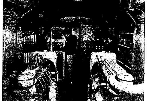
When the President travels by train he keeps in instantaneous touch with whatever may be going on, and the photo above explains how he does it. Shown is the interior of a former Pullman car converted into a communications center for the chief executive. Equipment includes generators, telephones, and a two-way phone for direct communication with the White House.
