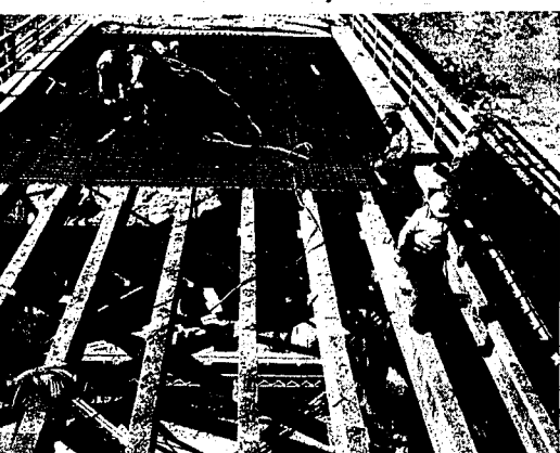
Tight rope walkers at the circus have the comforting thought that there's a net below, but steel workers at the 470-foot-high rim-to-rim bridge have no such solace. These workers appear as they prepared the way for laying of the new armoured steel decking, shown in background, and for the railing and walkways, which are rapidly moving out from the north side of the structure. This photo, was taken by John Brennan from a crane which swung him above the bridge. (Staff engraving)
