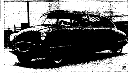
William B. Stoll, automotive and aviation engineer, sits at the wheel of the passenger car in Detroit which he has constructed of fiberglass plastic, except for the doors. There are many other unorthodox features, including engine in rear; no chassis or axles; extra-long wheelbase; and a roto-hub interior with no front or rear seats in the conventional sense. (AP wirephoto)
