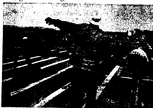
... and new steel deck goes into place
