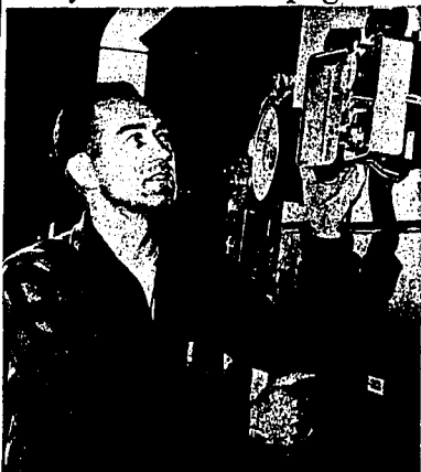
Lloyd E. Palmer, operator at the Idaho Power company sub-station, opens the case of the astronomical clock that automatically switches the city's street lights on and off. It adjusts itself to turn the lights on earlier during winter months, later during long summer days. (Staff photo—overright)
