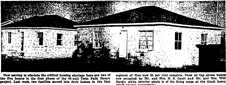
New project to alleviate the critical housing shortage here are the first of the homes in the first phase of the 40-home Twin Falls Homes project. Last week, two families moved into their homes in the first segment of five now 85 per cent complete.
