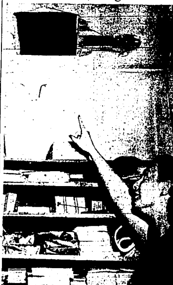
Marjorie Savelberg is shown above pointing to the hole through which vandals entered the Sears, Roebuck store here. A similar hole was cut in the roof by the vandals who climbed a telephone pole at the rear of the building to reach the roof. Miss Savelberg is an employee at the store. (Staff photo-photography.)
