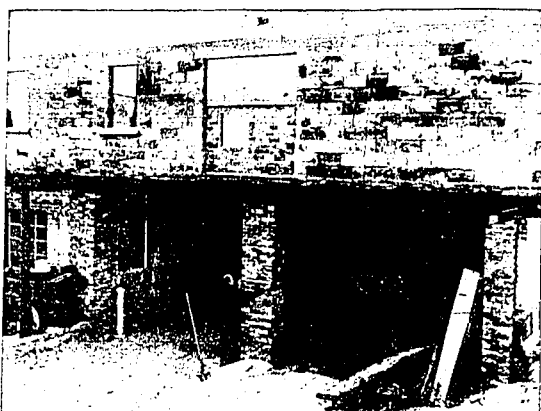
Clarence Booth, businessman of Lakewood, N. J., is building an atom-bomb-proof home. The house has one floor above ground and one floor below. It will be reinforced with tons of steel and concrete. It will be protected against atomic radiation by glass-like tile, and against poisonous gases by an air-proof locking door system.
