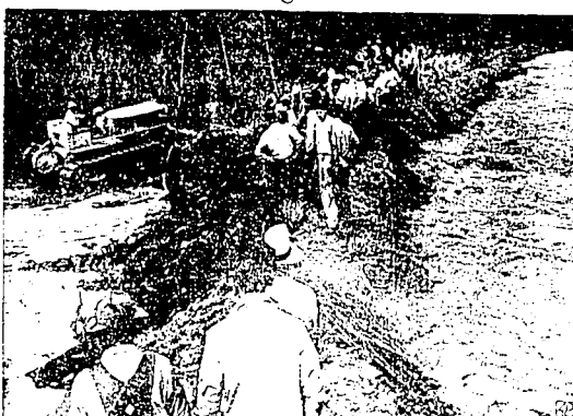
Workers, with the aid of a bulldozer, make hastily trailer a levee in the Yakima, Wash., area as they battle rising waters. Many were forced to flee their trailer homes near here. (AP wirephoto.)
