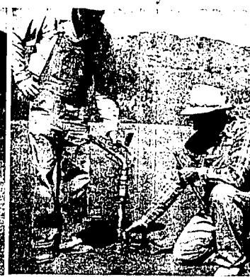
for the golf course, attaches one of the new high pressure sprinklers to a buried water main while Harold Oschner holds open the coupling cover. Lack of hose is one of the big advantages of the system. (Photos by Ronald J. Rice-staff engravings)
