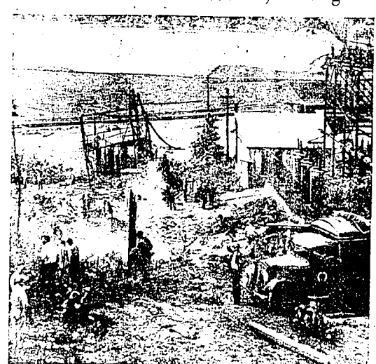
Charged hillside in eastern Pennsylvania is scene where DC-6 with 43 persons aboard struck a high tension line, then crashed into a transformer at power sub-station and exploded, throwing wreckage and bodies in every direction. The ill-fated flight, flying 30 feet off the ground, was attempting an emergency landing. All aboard were killed (NEA telephoto)
