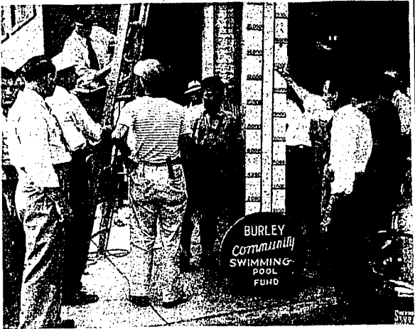
Members of the Burley Junior Chamber of Commerce are shown above as they erected a large thermometer at the intersection of Main street and Overland avenue to record progress of a drive to raise $50,000 for construction of a new swimming pool in Burley.
