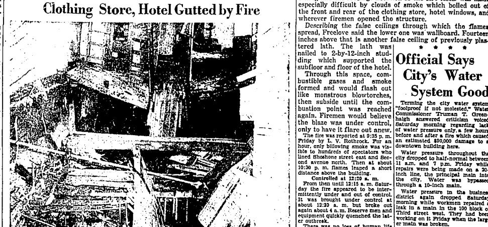
Shown above is a general view of damage caused in a three-hour fire Friday night at the Shirley-Mendiola Men's store and the Douglas hotel. At the top are two hotel rooms ready to fall into the store below. In the foreground are portions of the burning building which collapsed into the store. Shown in the picture above is the view of the Douglas hotel, South Carolina, and firemen working, lower right and left, cleaning debris from the furniture and fixtures in the hotel room at the upper right. (Photos by Ron Rice-staff engravings)
