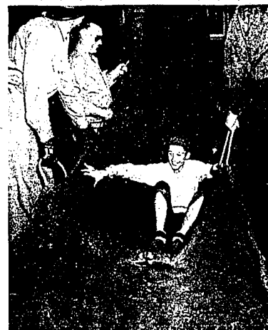
shown at the end of his slide down the evacuator. When set up, the device is similar to any playground slide. Fire Chief E. H. Freecove and school officials will use the test in trying to determine a means of eliminating the fire hazard in the school's dome. The dome is presently used for music classes. (Staff photo-engravings)
