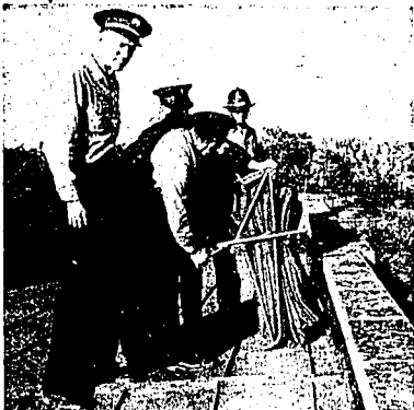
Members of the Twin Falls fire department are shown at left clamping the evacuator canvas fire escape to the roof of the Twin Falls high school directly in front of the school dome.
